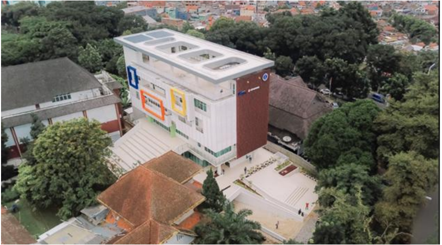
Gambar 7.13. Contoh Bangunan Technp Park ( Science Techno Park (STP) ) ITB Bandung
