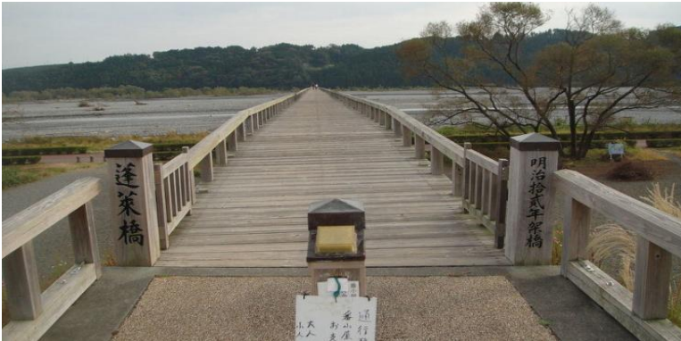
Gambar 1.4. Jembatan Horai Bridge (Hendara, 2017)
