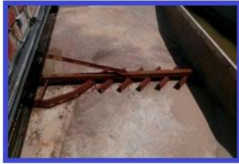
Gambar 1.3 Showing the inner view of grit removal Sumber : (Salvi and Patil, 2021)
