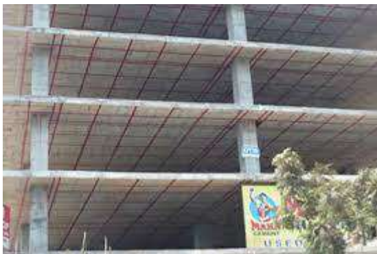
Gambar 4.24. Plat post-tensioned (Sumber : uconpt.com, 2024)
