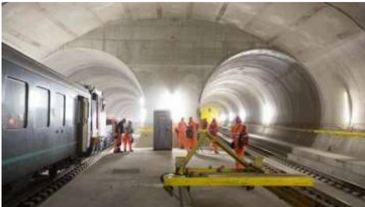
Gambar 4. 3. Proyek Terowongan Gotthard Base Tunnel, Swiss (Sumber : Tribun Kaltim, 2016)
