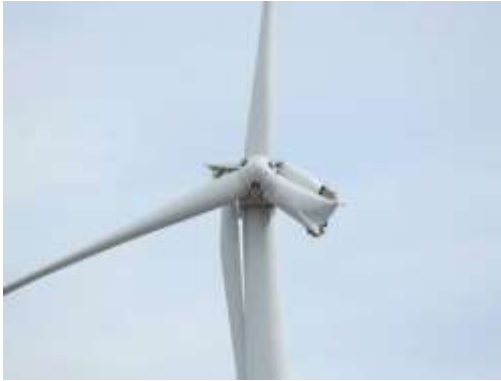
Gambar 8.8 : Kerusakan turbin akibat over-speed
