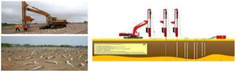
Gambar 6.1. Skema Dan Penerapan Prefabricated Vertical Drains ( James D. Hussin, 2006)
