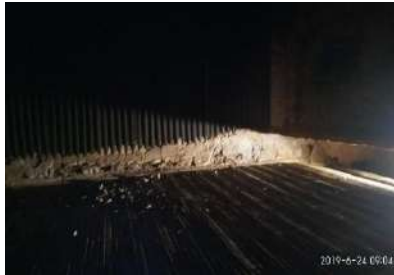
Gambar 3. 6. Inspeksi Refractory Boiler #2
